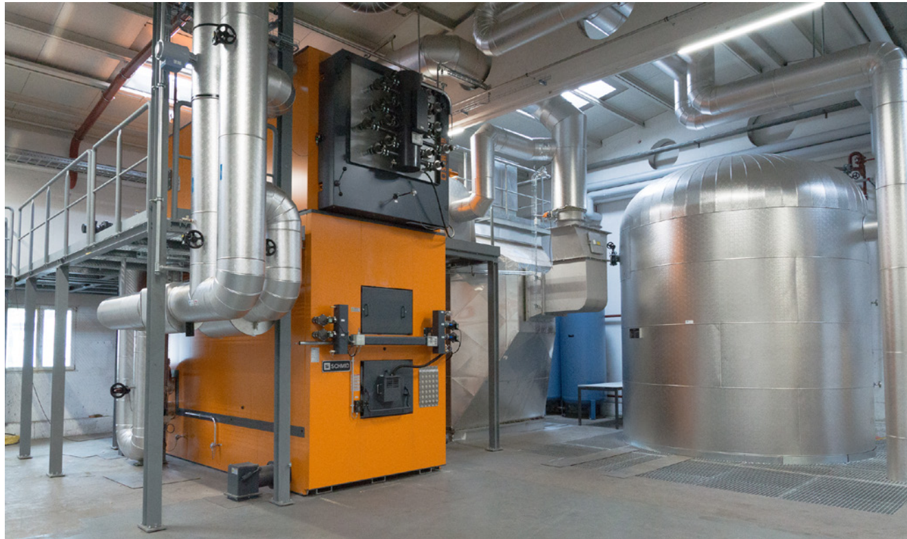
Schmid - Moving grate boiler UTSR-1600 visio
