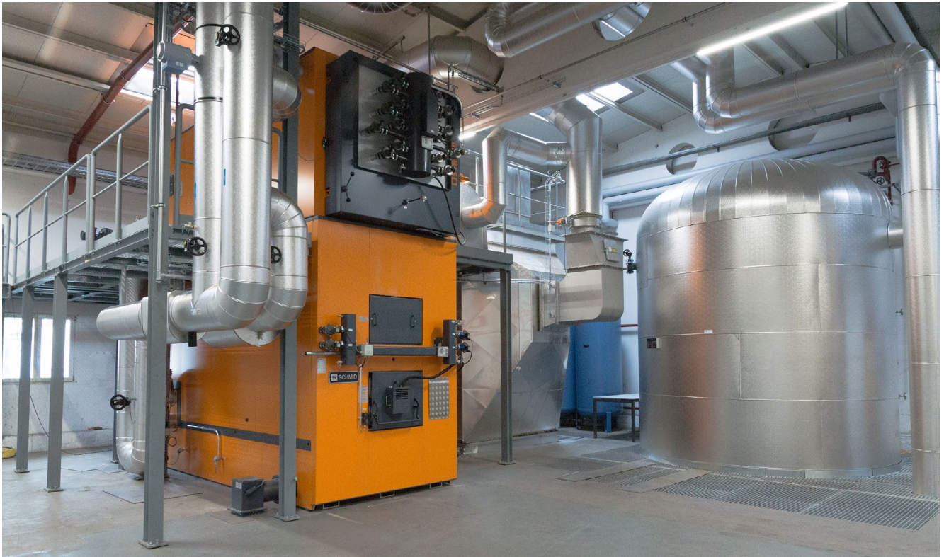
Schmid Mawera Group - Moving grate boiler UTSR-1600 visio
